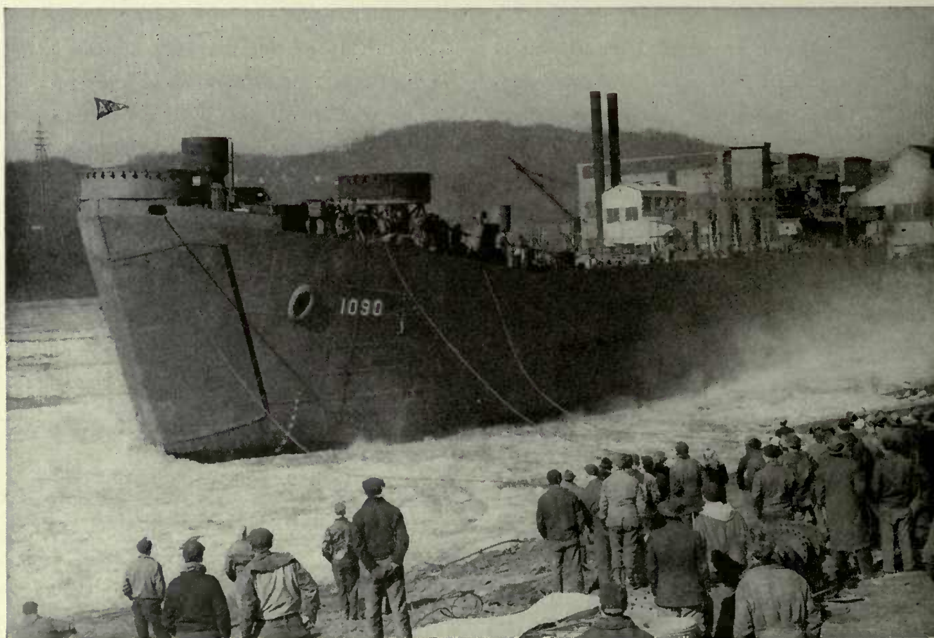
U. S. Steel built 119 LST's—Landing Ships, Tanks—and reduced construction time from 260 to 63 days.
